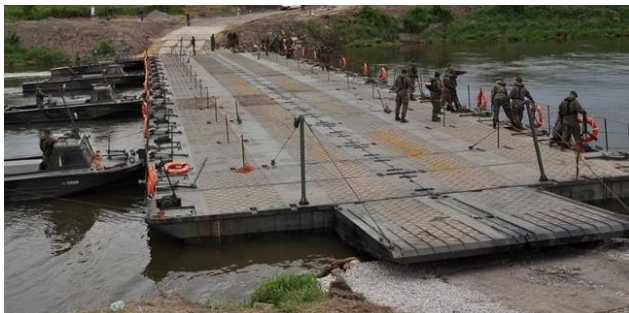
Fig.1. Polish ribbon pontoon bridge PP-64 [10]
