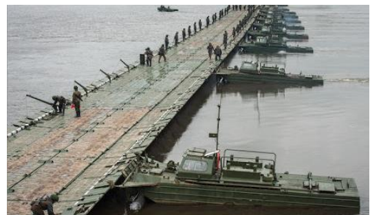
Fig.4. Russian ribbon pontoon bridge PP-2005 [13]
